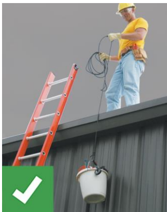
RIGHT Haul materials with a line rather than carry them up an extension ladder. Use extra caution when carrying anything on a ladder.
