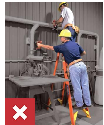
WRONG DON'T exceed the maximum load capacity or duty rating of a ladder. DON'T permit more than one person on a single-sided stepladder
